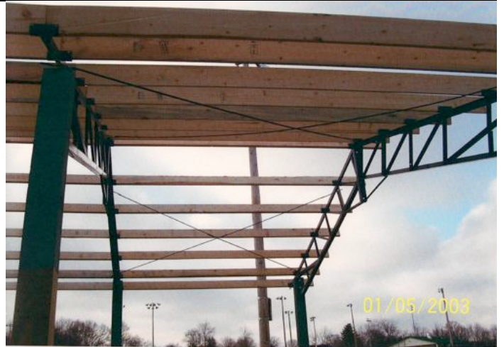
Post Frame/Metal Truss Bracing
