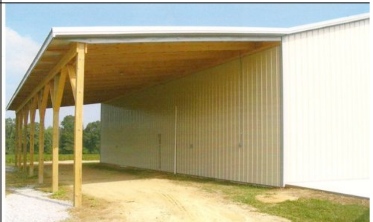
Wood Rafter Side Shed
